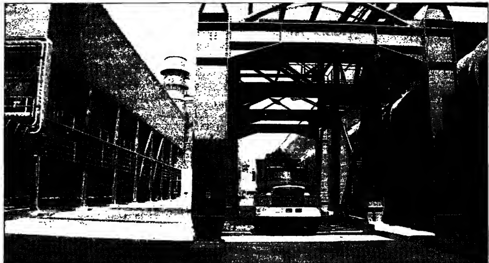
Gas-clearing plant and solid-bath unloading station for the new No. 4 potline.
